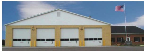
Attica Township Fire Station
